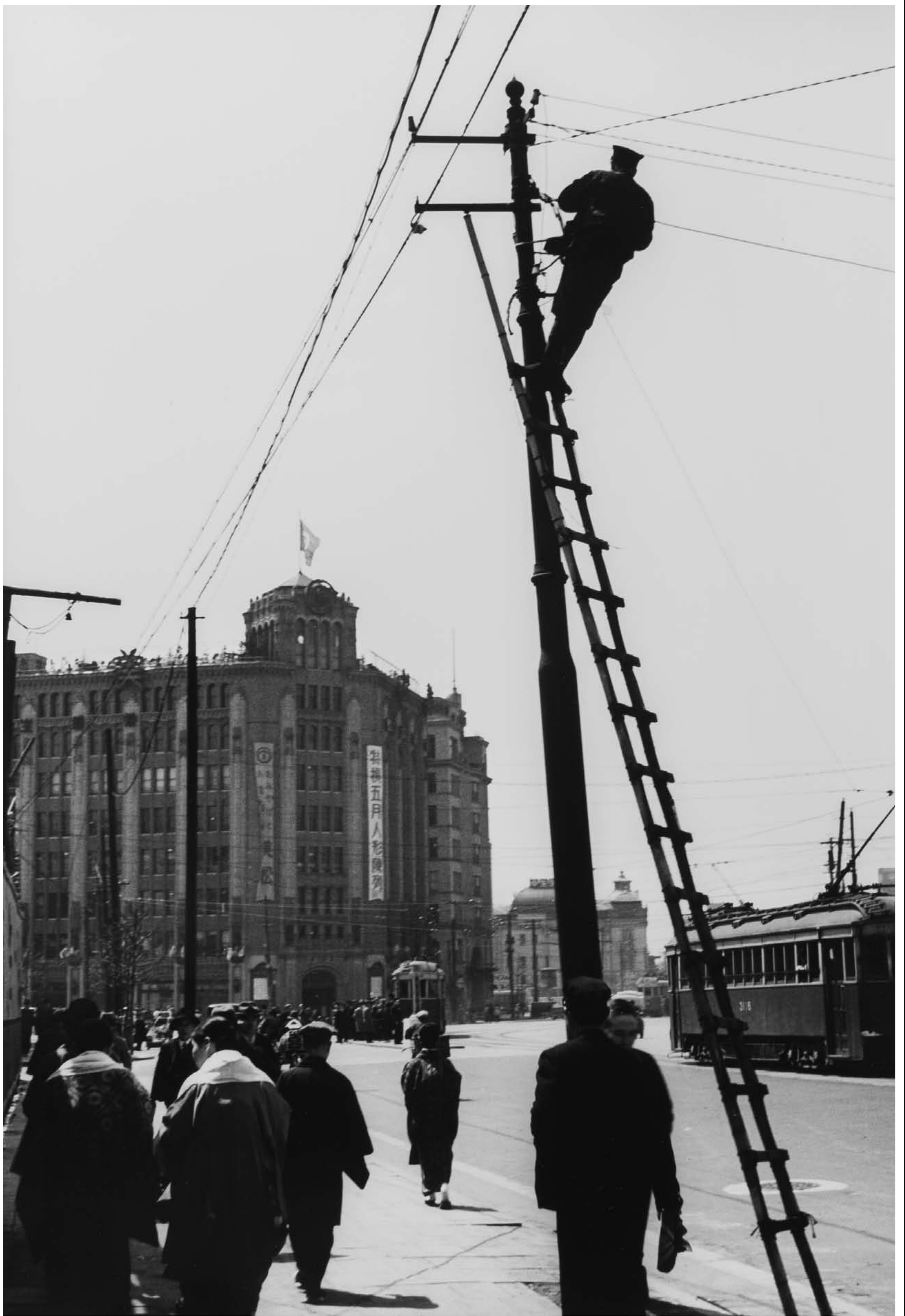
TSM 32 Fixing an electricity pole in front of Ueno Station 1936
